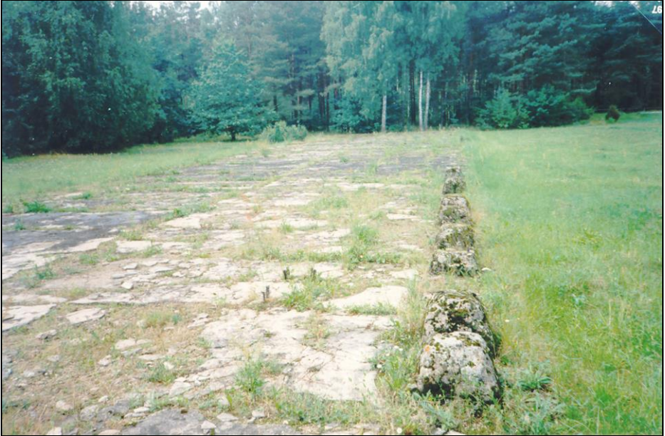
Photo 9: Treblinka I. One of the eight concrete foundations, on which the barracks stood. © Carlo Mattogno, 1997.
