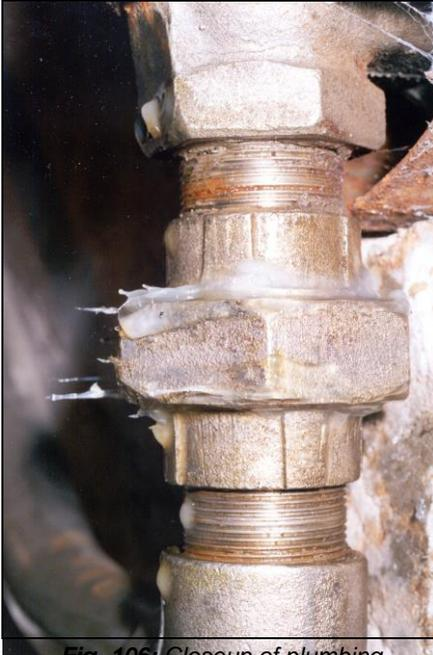
**Fig. 106:** Closeup of plumbing underneath the gas chamber covered in Vaseline to indicate leaks.
