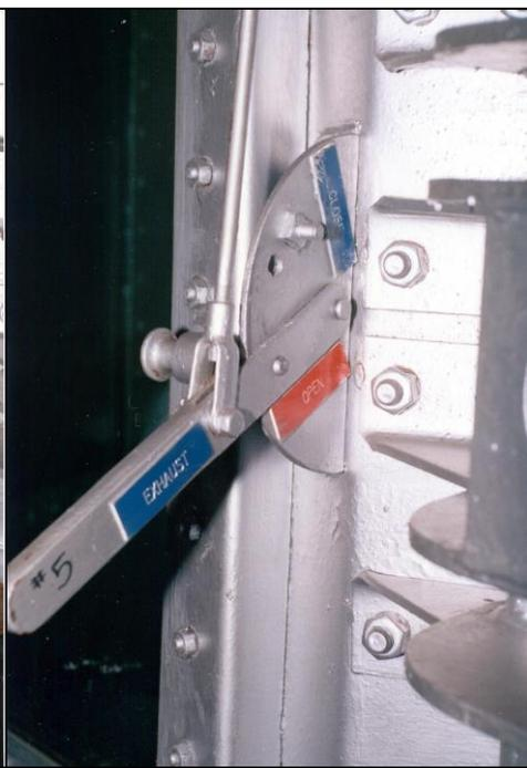
**Fig. 99:** Closeup of lever used to open and close exhaust stack.
