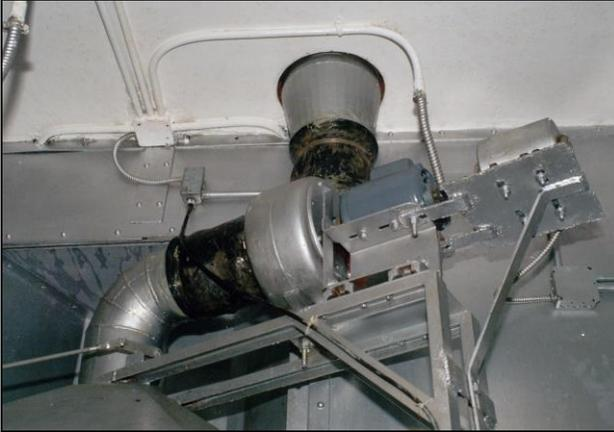
**Fig. 102:** Exhaust fan and stack on top of gas chamber.
