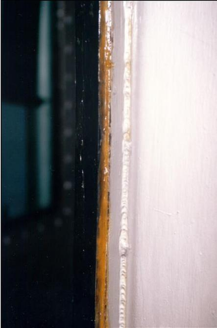
**Fig. 104:** Closeup of rubber seal around gas chamber door, also covered in Vaseline when in use.
