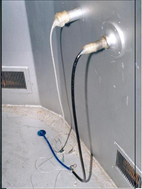
**Fig. 111:** Inside gas chamber where stethoscope and other body monitoring line enter. They are covered in Vaseline to indicate leaks. Fresh air vents on the walls close to the floor.
