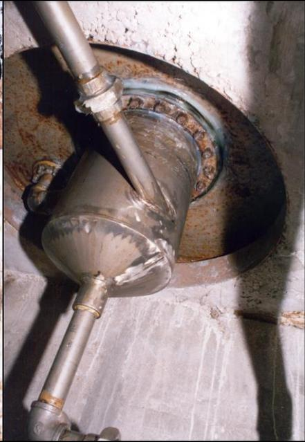
**Fig. 107:** View of stainless-steel plumbing and chemical container directly under seat in gas chamber.
