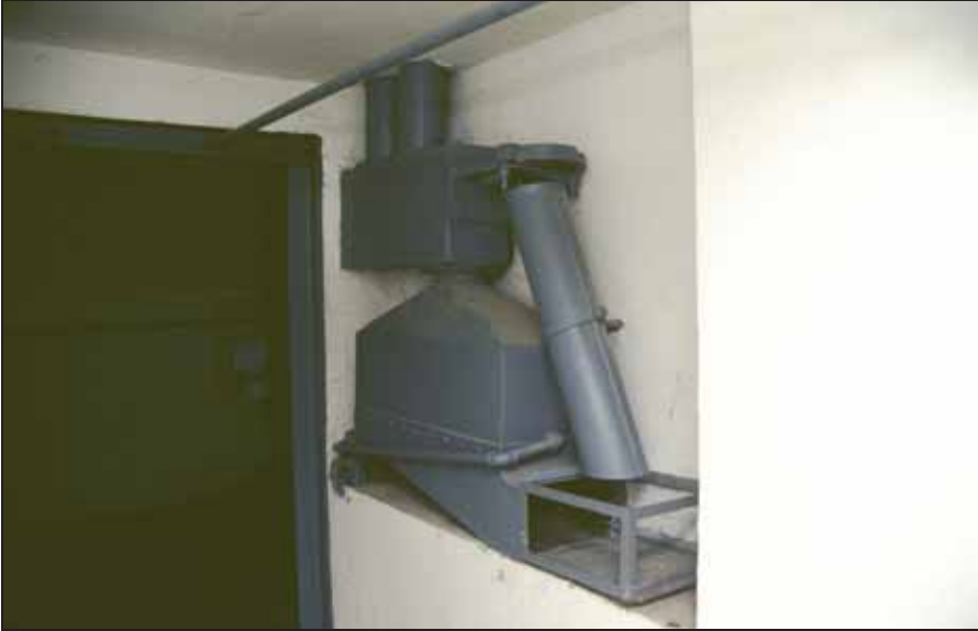
Illustration 21: The inside of one of the four Degesch delousing chambers as it can be seen today in Dachau. At the top the can opener controlled from the outside. The Zyklon pellets slide through the pipe into a wire-mesh basket at the bottom, through which warm air is conducted by the heater/fan unit (below the can opener).
