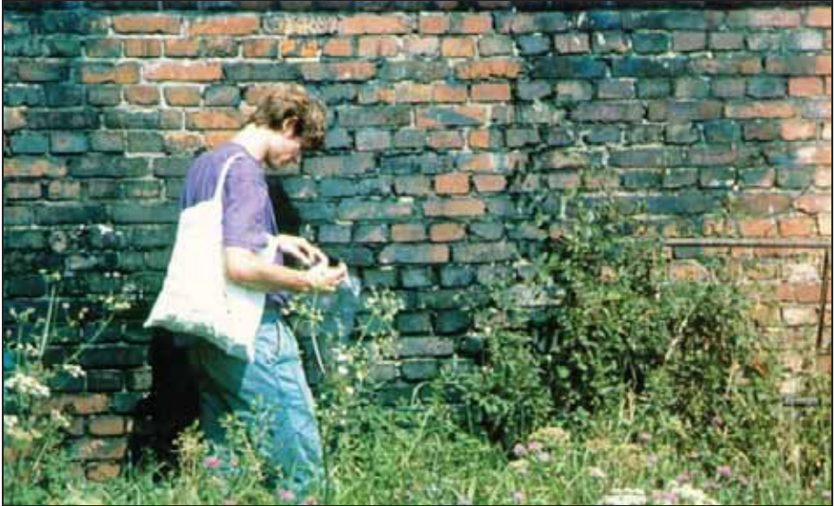
Illustration 18: Gernar Rudolf noting the blue hue of a delousing chamber at Auschwitz-Birkenau (building no. BW 5b)
