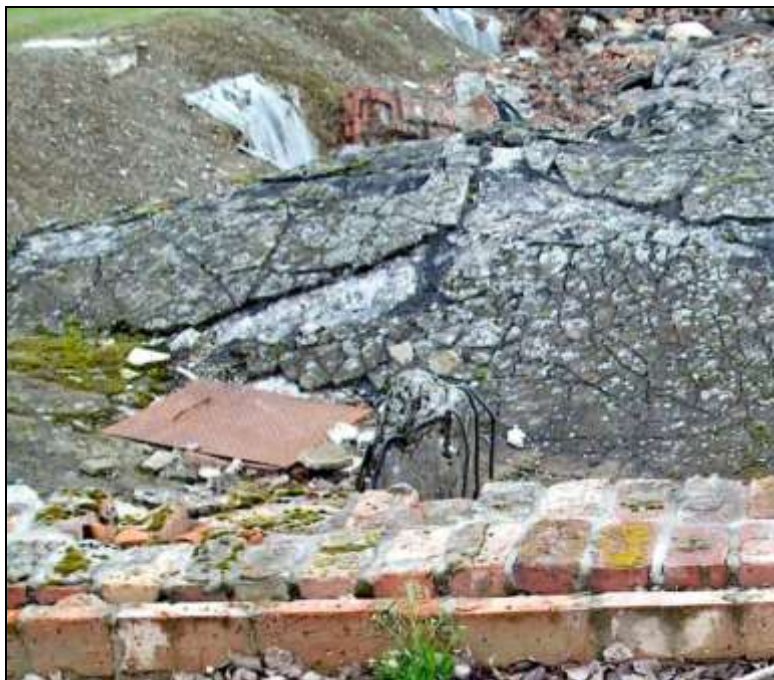
Photo 10: Steel lid of an inspection port on the roof of Morgue #2 of Crematorium II in Birkenau. © C. Mattogno.
