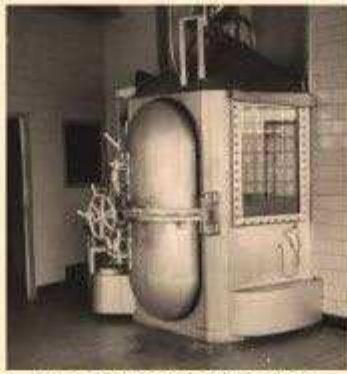
Gas chamber door, Colorado
