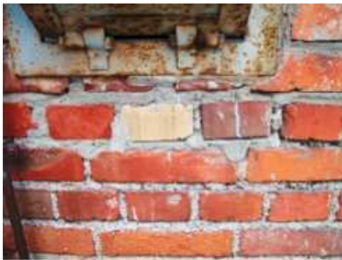
Photo 18: Mortar variation in right chute.
