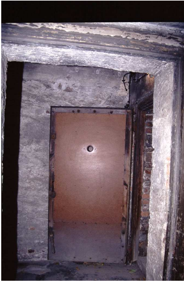
Illustration 4: Make-shift air-raid-shelter door of Krematorium I made of wood with a thin sheet metal cover, probably built by inmates in the camp's workshop.
