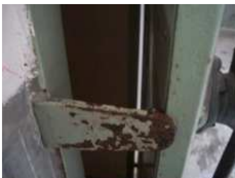
Photo 10: Exit door obstruction.
