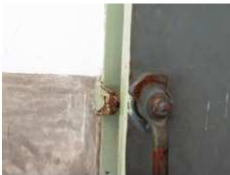
Photo 9: Exit door obstruction.
