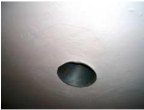
Photo 7: Rework to ceiling around shower head.
